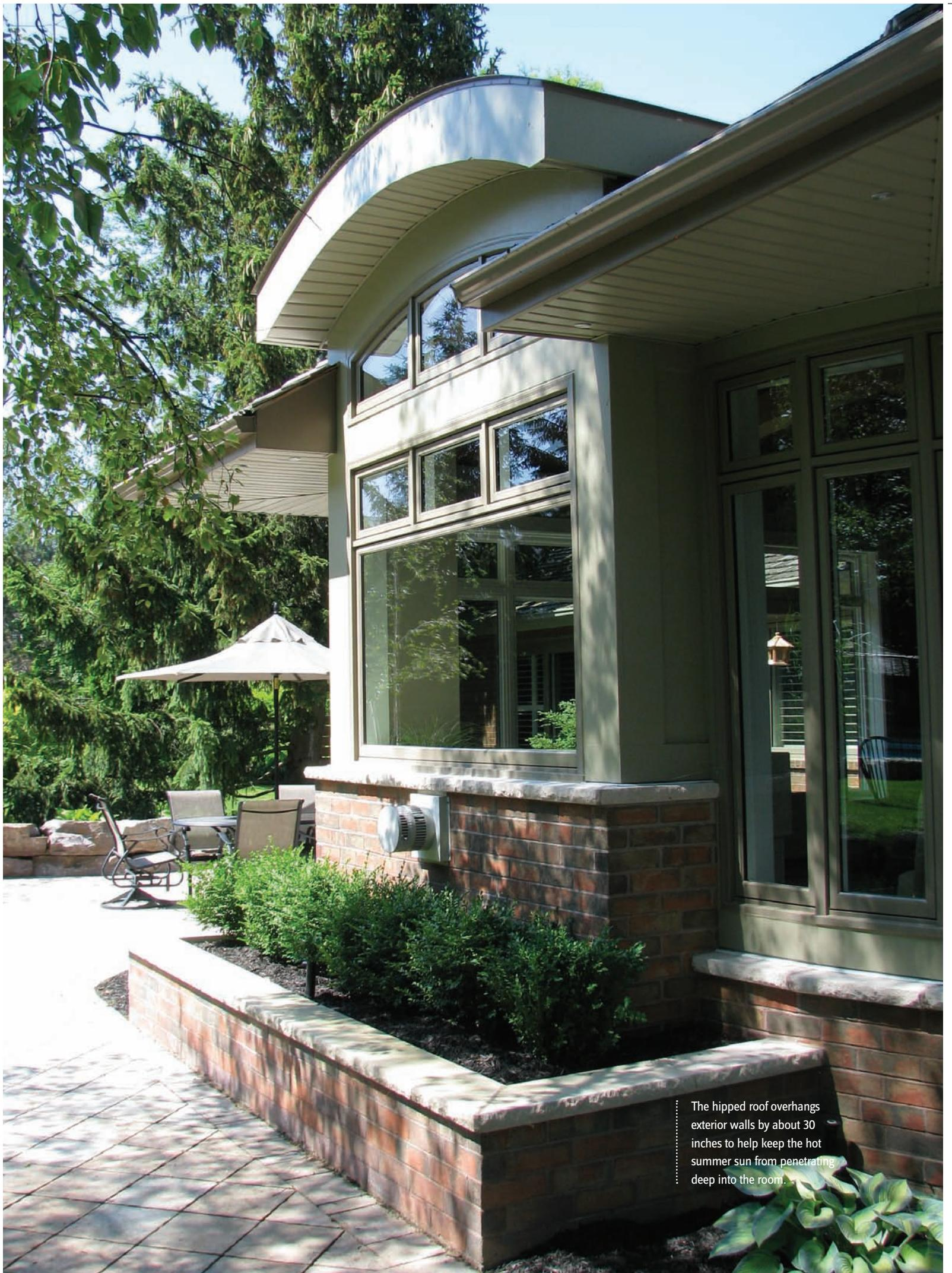
The hipped roof overhangs exterior walls by about 30 inches to help keep the hot summer sun from penetrating deep into the room.
